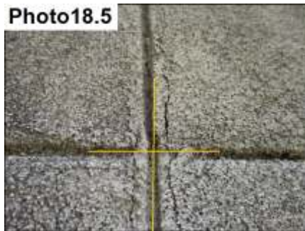
Control Joint Cracks/ Seal And Paint
