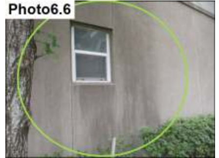
Mildew And Run-Off Stains/ Seal
