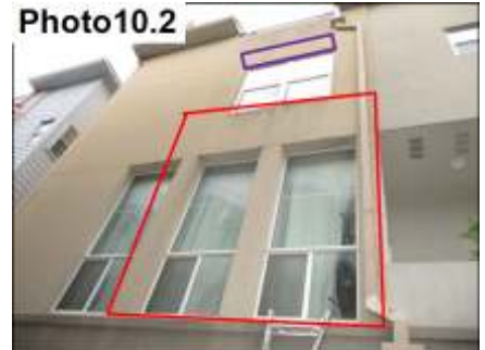
Confirmed Substrate And Potential Frame Damage/ Repair/Add Relief
