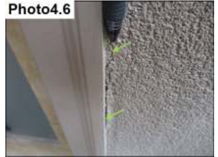
Door Trim And Miter Sealants/ Seal
