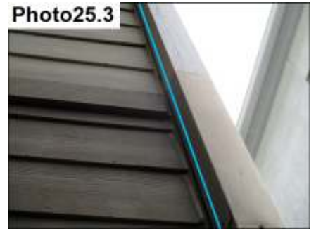
Siding Trim/Stucco Termination Sealants/ Seal
