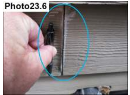
Siding Sealants/ Seal
