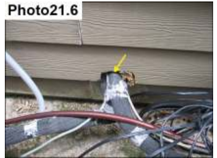
Penetration Sealants/ Seal
