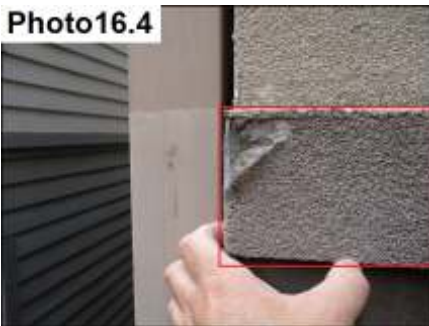
Broken Accent Band/ Repair And Seal
