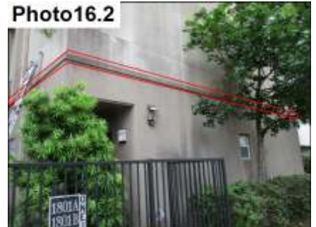
Broken Accent Band/ Repair And Seal
