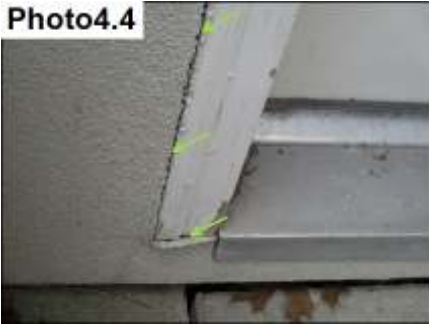
Door Trim And Miter Sealants/ Seal
