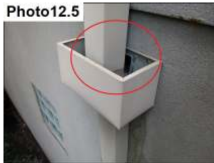
Scupper Sealants Missing / Seal
