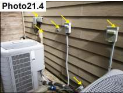
Penetration Sealants/ Seal
