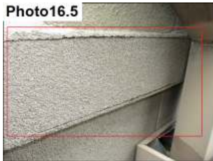
Broken Accent Band/ Repair And Seal
