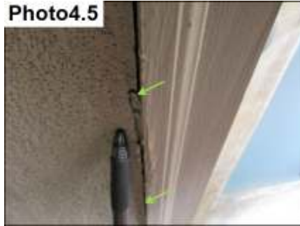
Door Trim And Miter Sealants/ Seal
