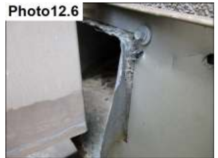
Scupper Sealants Missing / Seal
