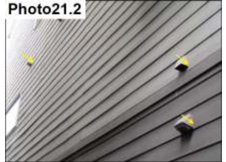
Penetration Sealants/ Seal
