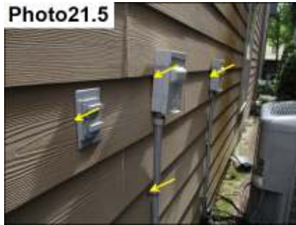
Penetration Sealants/ Seal
