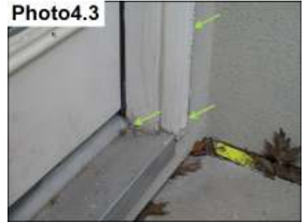
Door Trim And Miter Sealants/ Seal
