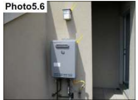
Penetration Sealants/ Seal
