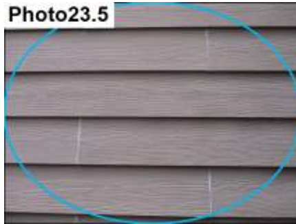
Siding Sealants/ Seal
