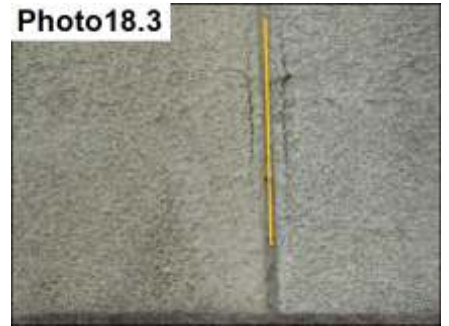
Control Joint Cracks/ Seal And Paint
