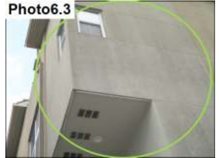
Mildew And Run-Off Stains/ Seal
