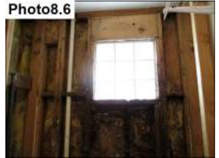
Confirmed Substrate And Frame Damage/ Repair
