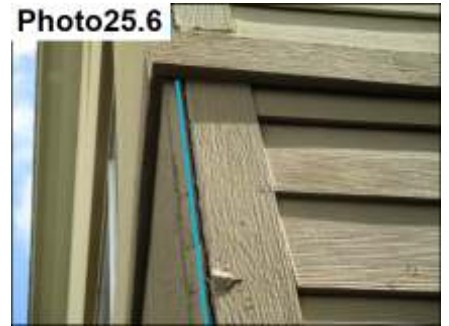
Siding Trim/Stucco Termination Sealants/ Seal
