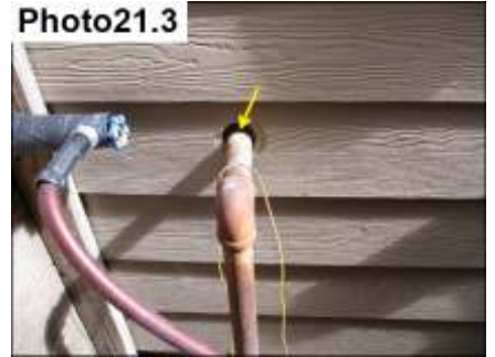
Penetration Sealants/ Seal
