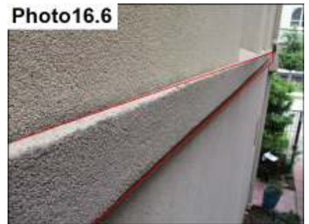
Broken Accent Band/ Repair And Seal
