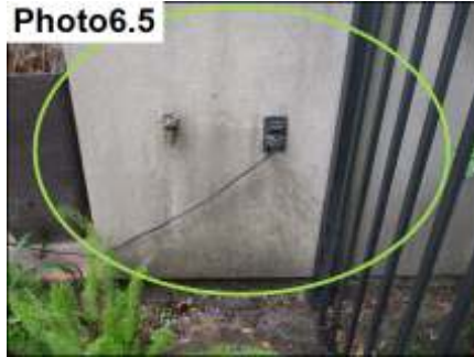
Mildew And Run-Off Stains/ Seal
