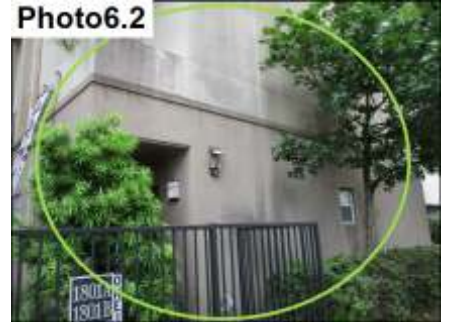
Mildew And Run-Off Stains/ Seal
