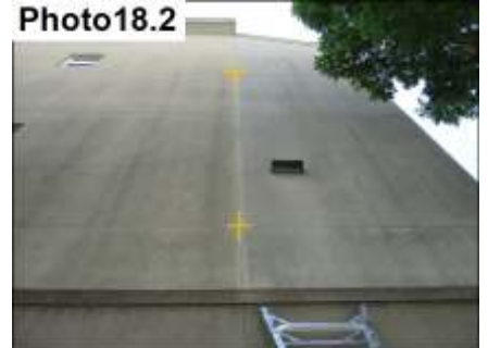
Control Joint Cracks/ Seal And Paint
