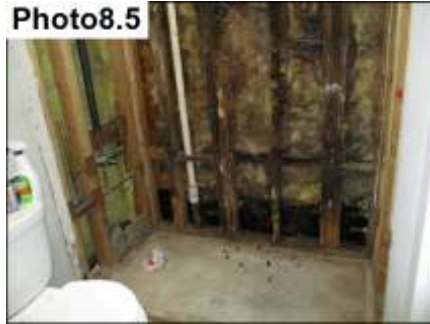
Confirmed Substrate And Frame Damage/ Repair
