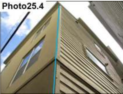
Siding Trim/Stucco Termination Sealants/ Seal
