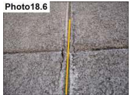
Control Joint Cracks/ Seal And Paint
