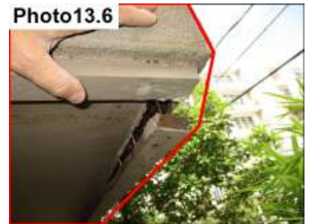
Confirmed Substrate And Potential Frame Damage/ Repair
