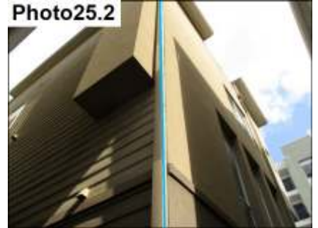
Siding Trim/Stucco Termination Sealants/ Seal
