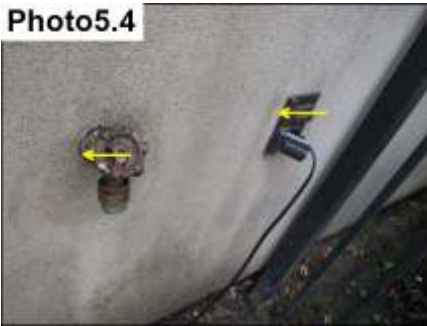
Penetration Sealants/ Seal
