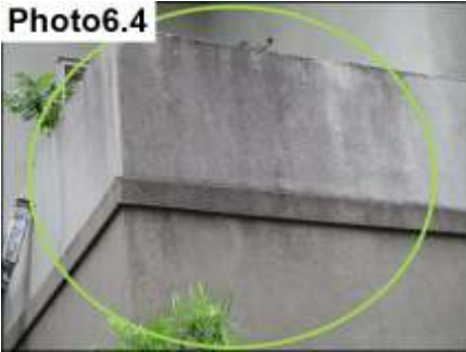
Mildew And Run-Off Stains/ Seal
