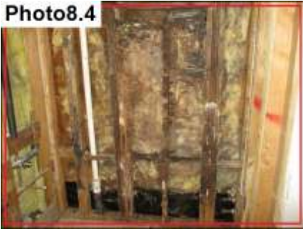
Confirmed Substrate And Frame Damage/ Repair
