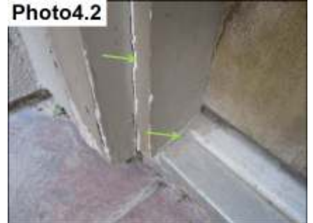
Door Trim And Miter Sealants/ Seal
