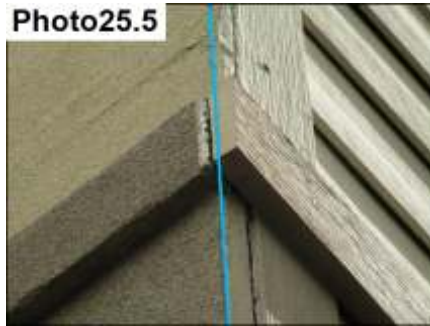
Siding Trim/Stucco Termination Sealants/ Seal
