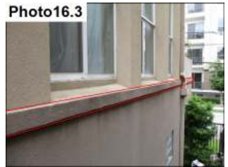
Broken Accent Band/ Repair And Seal
