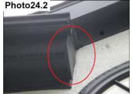
Roof Diverter Flashing Sealants/ Seal
