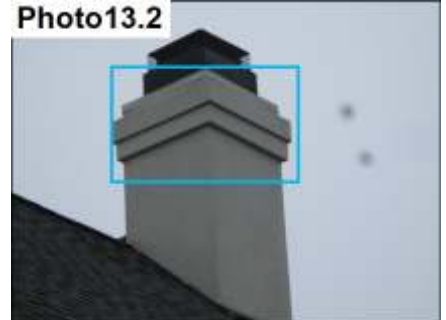
Chimney Cap Present/ Seal Metal Cap/Accent Termination
