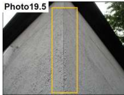
Cracks/ Repair
