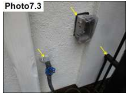
Penetration Sealants/ Seal
