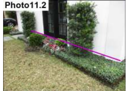
Stucco In Close Proximity To Grade/ Pull Back
