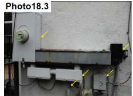
Penetration Sealants/ Seal
