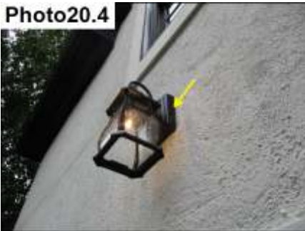
Penetration Sealants/ Seal
