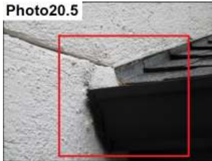
Missing Kickout Flashing/ Modify
