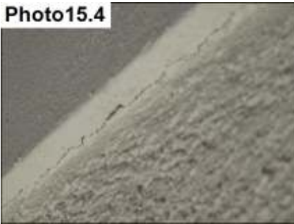
Accent Band/Stucco Termination Sealants/ Seal
