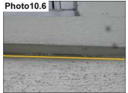
Accent/Stucco Termination Sealants/ Seal
