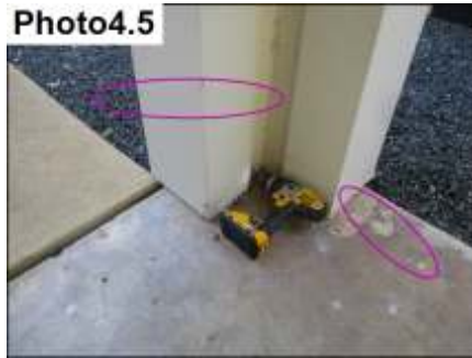
Substrate Damage /Repair
