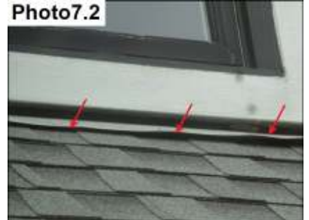
Roof Penetration/ Re-Fasten And Seal
