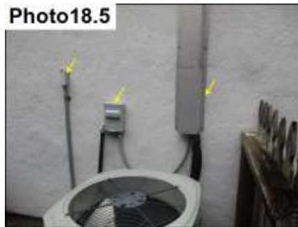
Penetration Sealants/ Seal
