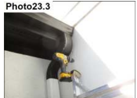
Missing Kickout Flashing/ Modify
