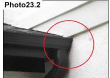
Missing Kickout Flashing/ Modify
