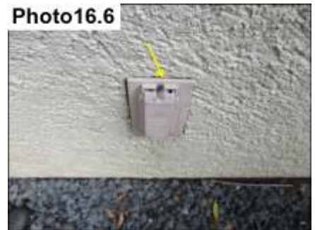
Penetration Sealants/ Seal
