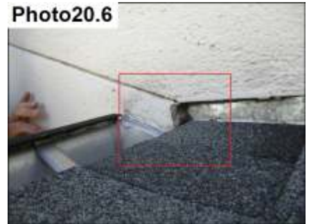
Missing Kickout Flashing/ Modify
