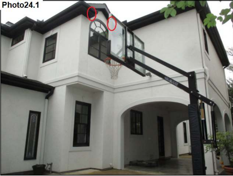
Roof Diverter Flashing Sealants/ Seal
