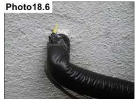
Penetration Sealants/ Seal
