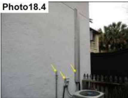
Penetration Sealants/ Seal
