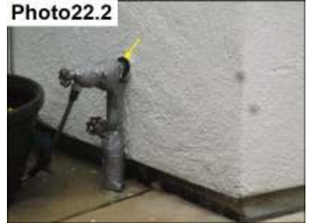
Penetration Sealants/ Seal
