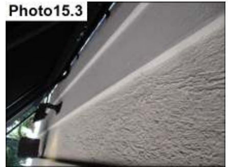
Accent Band/Stucco Termination Sealants/ Seal
