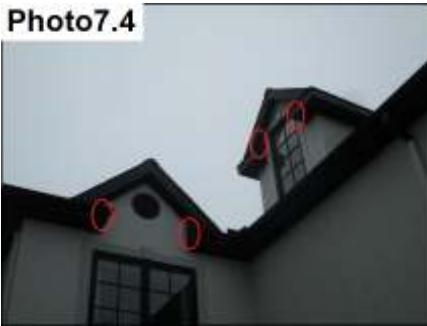
Roof Diverter Flashing Sealants/ Seal
