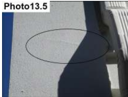
Previously Sealed Minor Crack/ Positive Detail
