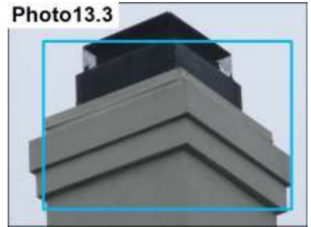
Chimney Cap Present/ Seal Metal Cap/Accent Termination
