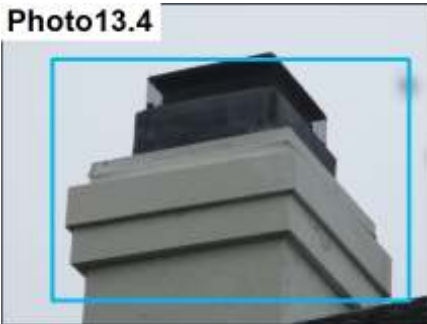
Chimney Cap Present/ Seal Metal Cap/Accent Termination
