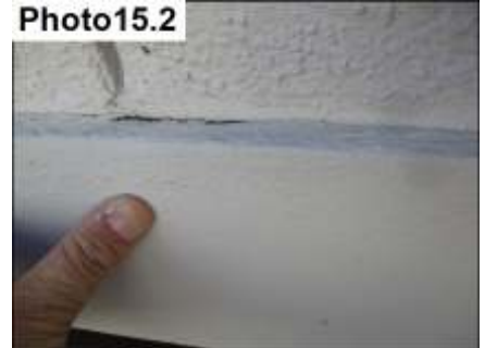
Accent Band/Stucco Termination Sealants/ Seal
